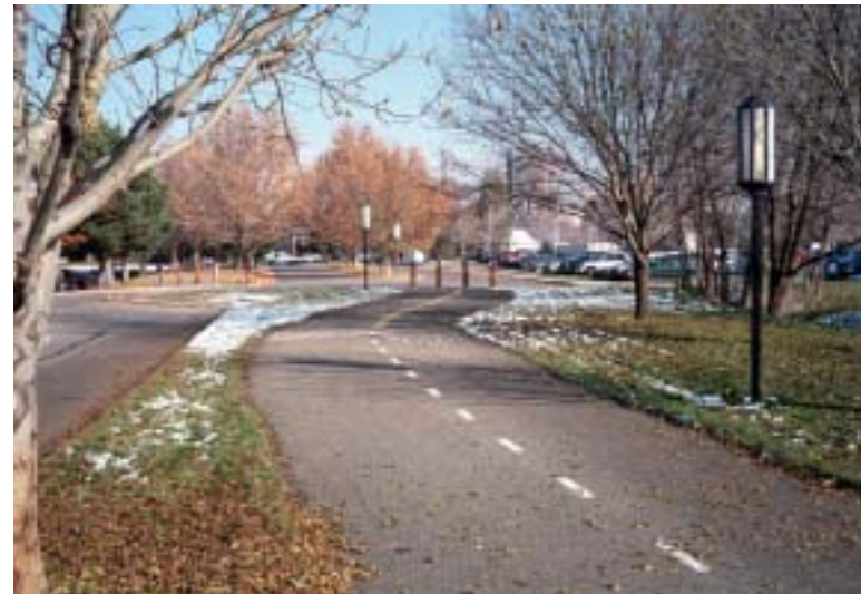
Pathway looking north at river
