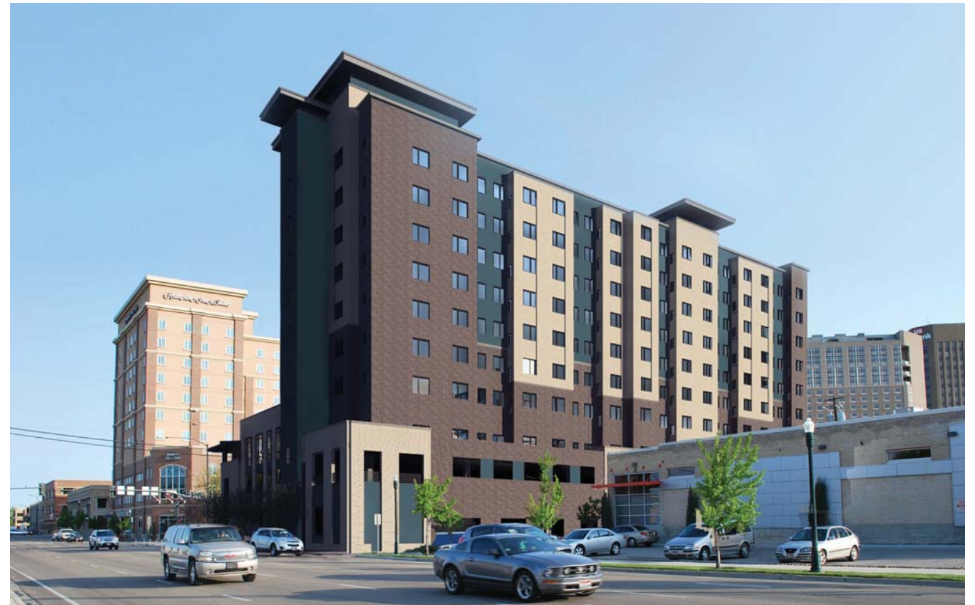
VIEW LOOKING WEST ON MYRTLE STREET
