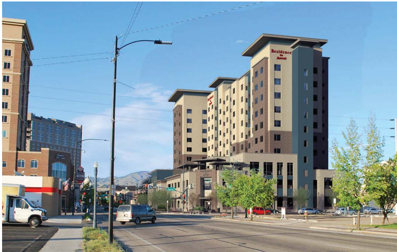
VIEW LOOKING NORTH ON CAPITOL BLVD.
