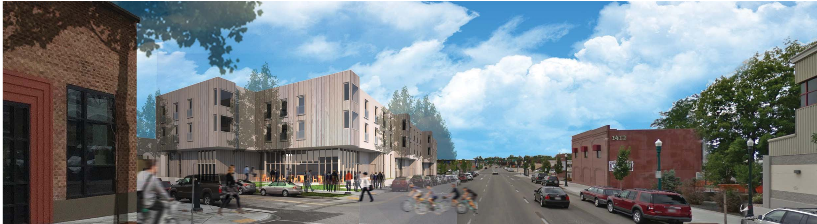
CONTEXT LOOKING WEST ON IDAHO STREET
