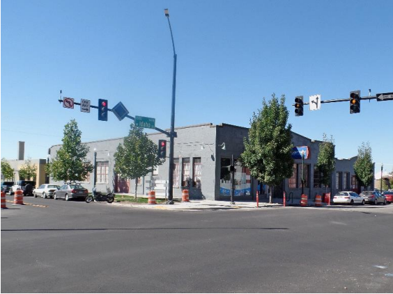
Subject site (improvements to be razed)
