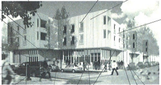
KAWNEER TRIFAB 451 FRONT GLAZED STOREFRONT BLACK MULLIONS CLEAR GLASS OR IPE SIDING VERTICAL 1X4 WHITEWASHED
