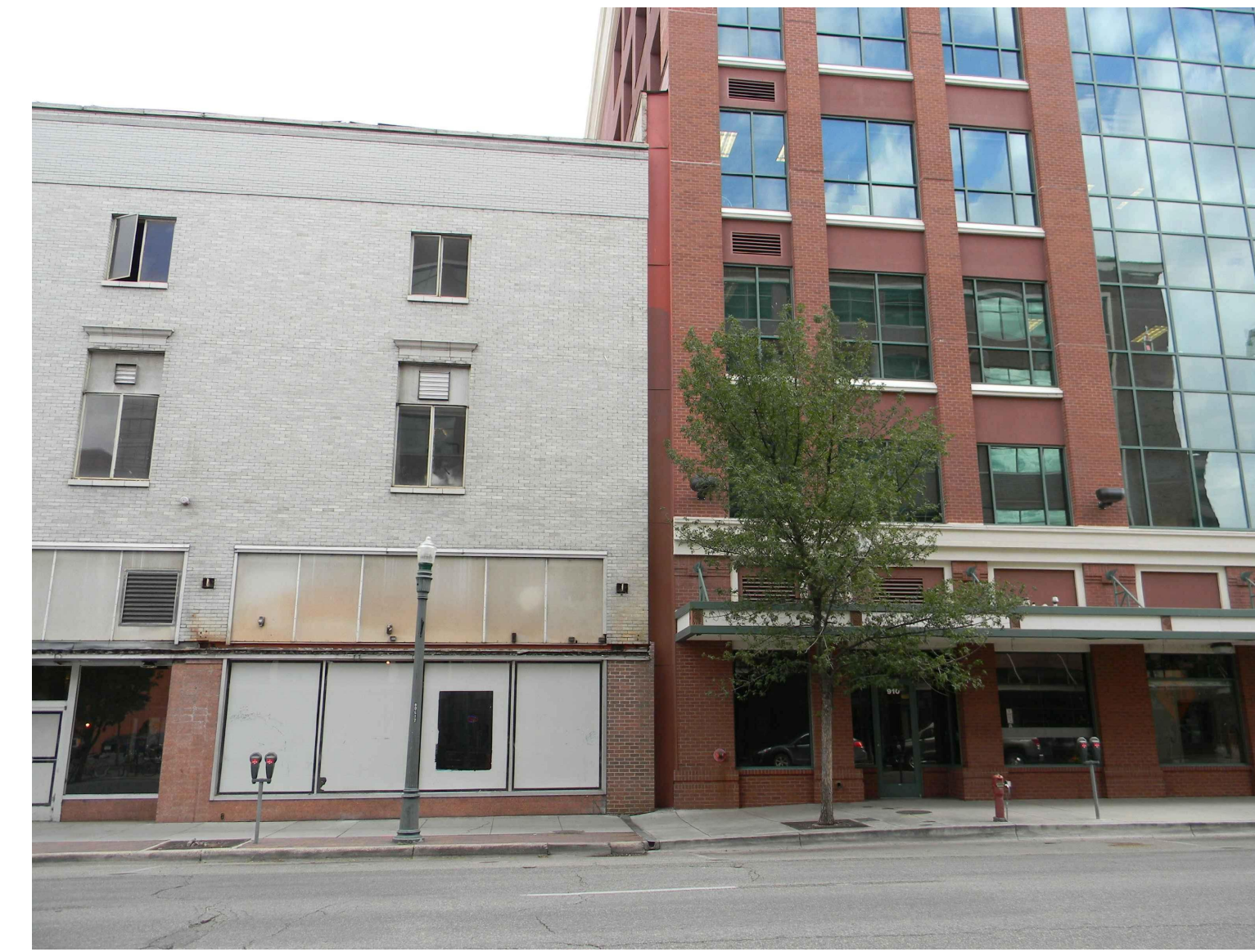
IDAHO STREET FACADE
