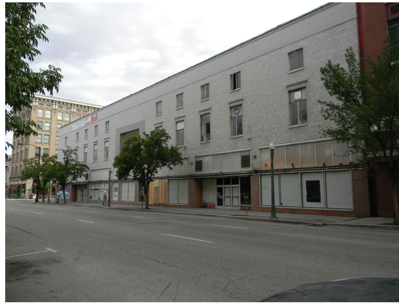
IDAHO STREET FACADE
