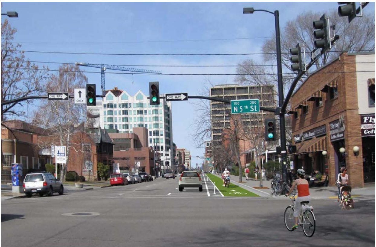
Figure 2: Parking Protected Bike Lanes (Idaho at 5 th )
