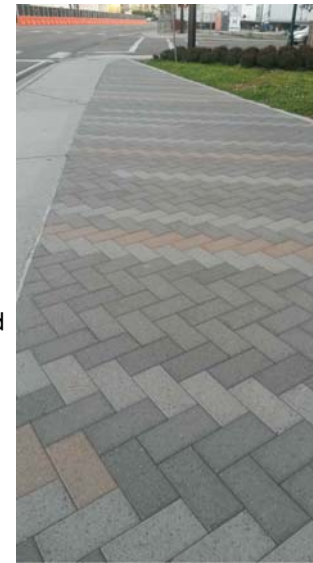
8 Pioneer Corridor Paving
