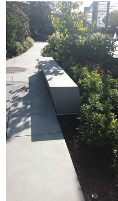
4 Concrete Seat Wall
