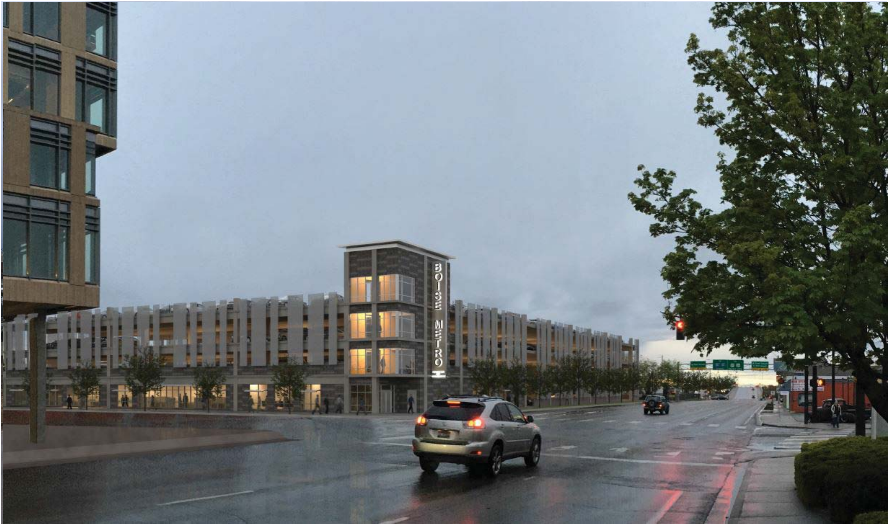
GARAGE VIEW FROM FRONT & 11TH STREET
