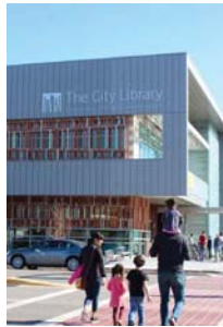
Clockwise from top left: Eccles Theater, Salt Lake City, UT; The City Library - Marmalade Branch, Salt Lake City, UT; Kunsthaus (Cultural Center) Weiz, Weiz, Austria.
