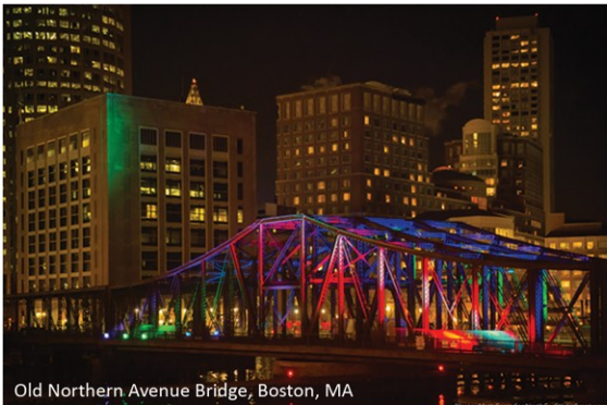
Old Northern Avenue Bridge, Boston, MA
