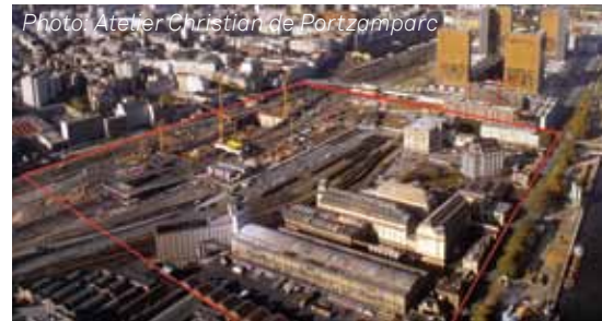
Photo: Atelier Christian de Portzamparc Aerial view of the Massena district before development
