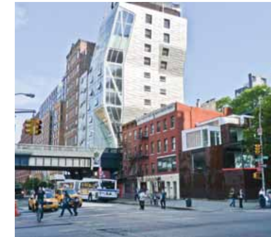
Selective redevelopment on existing footprints allows densification while preserving the grain of the walkable district. New York City, USA.
