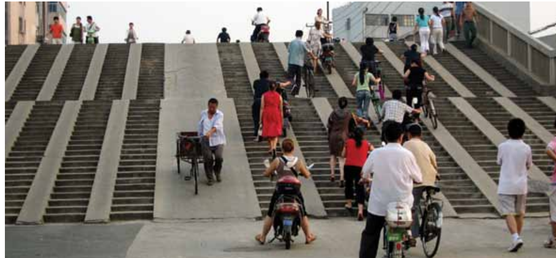
Simple interventions, like adding a ramp to stairs for people using cycles, make crossing more convenient. Changzhou, China.
