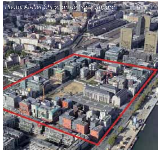
Photo: Atelier Christian de Portzamparc ... and during construction.
