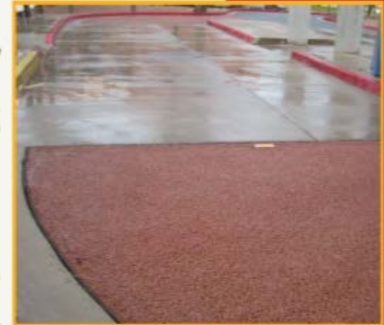
Pervious concrete allows for much faster water drainage. Above, the portion of ordinary concrete in Lot 9 is more wet than the pervious concrete in the foreground.
