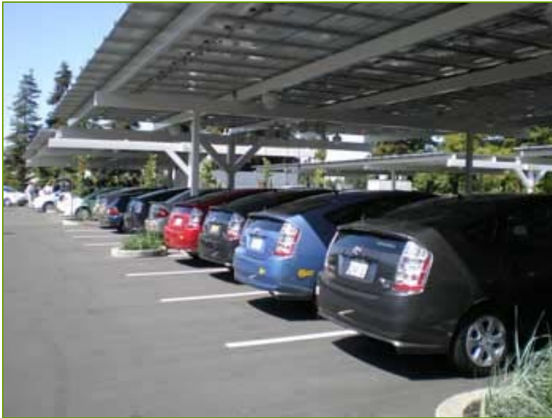
Canopies reduce heat island effect & provide sun and hail protection
