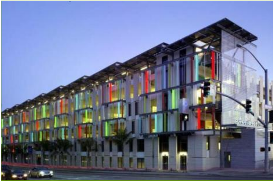
Santa Monica Civic Center Parking Solar panels at roof top canopies and on façade panels
