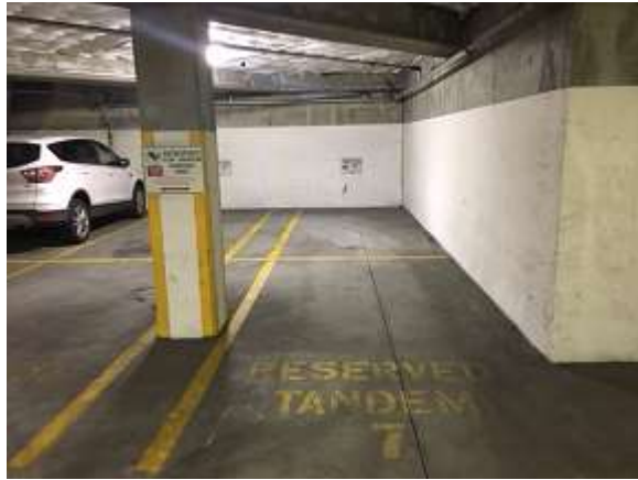
Row 7 tandem not effectively used due to wall
