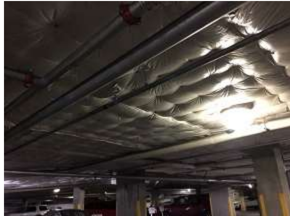
Interior ceiling view
