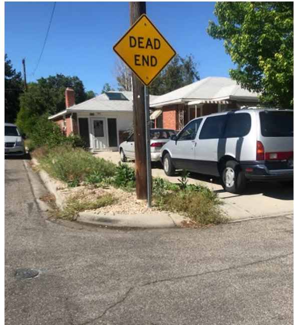
Dead end sign on Corporal Street, at the intersection of Corporal Street and North Stanley Street, facing north. Lack of street connectivity leads to inadequacies in the transportation network. Also visible in the photo is a lack of sidewalks on both streets, forcing pedestrians to walk in the street.
