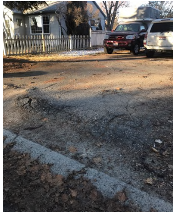
Buckling driveway along South Berkeley Street
