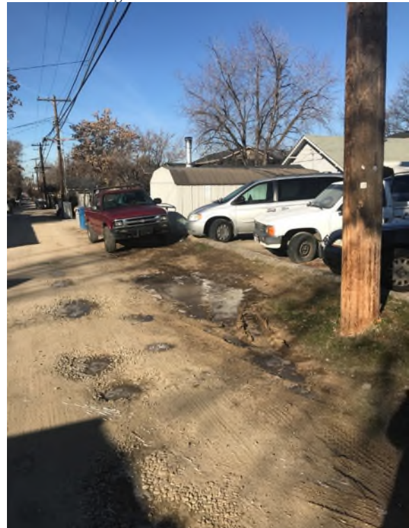
Unpaved dirt alley between Rose Hill Street and West Grover Street west of South Latah Street showing deterioration from wet and icy weather.
