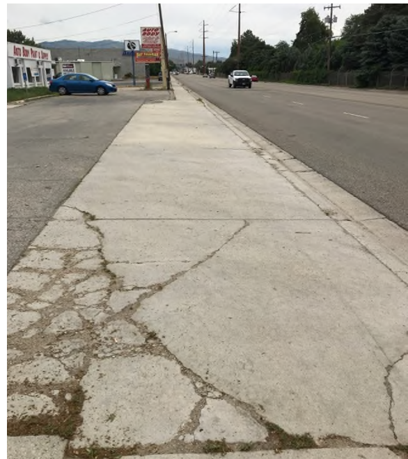
Deteriorated sidewalk on West Overland Road between South Wilson Street and South Orchard Street. At right, the sidewalk slopes to the gutter, providing a long and continuous driveway to the site at left, which is unsafe for pedestrians.
