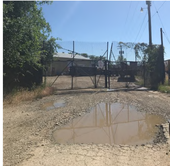
Entrance along West Gage Street showing inadequate drainage, cracked and deteriorated pavement, overgrowth of vegetation, and fence in disrepair.
