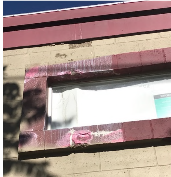
Deterioration and leaching of concrete on West Franklin building due to water.
