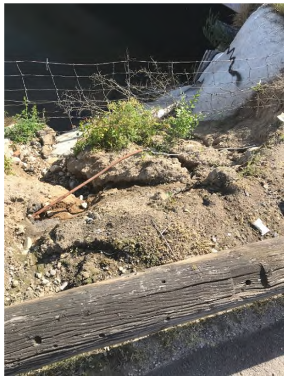
Canal opening along South Vista Avenue. Wire fence is an inadequate barrier to entry, creating an unsafe condition. The bottom picture shows a rusted protruding piece of rebar, which creates an injury risk.
