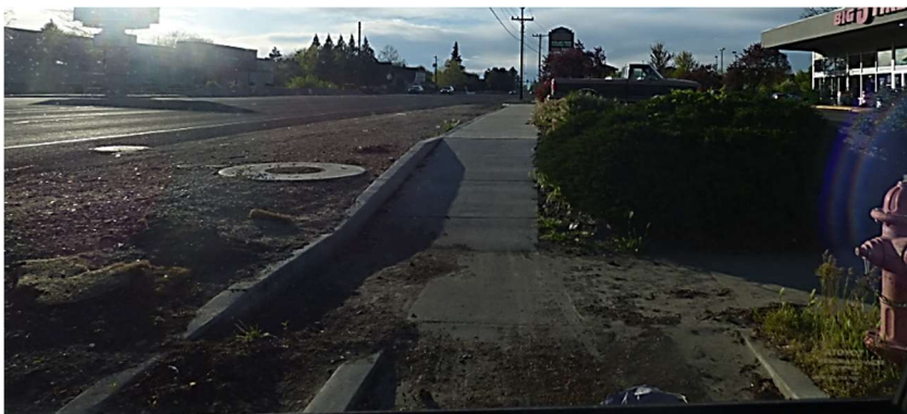
Badly deteriorated street margin, no curb/gutter; sidewalk area used for truck parking
