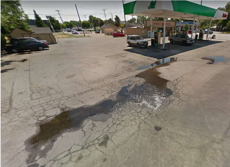
Parking surface deterioration and poor drainage
