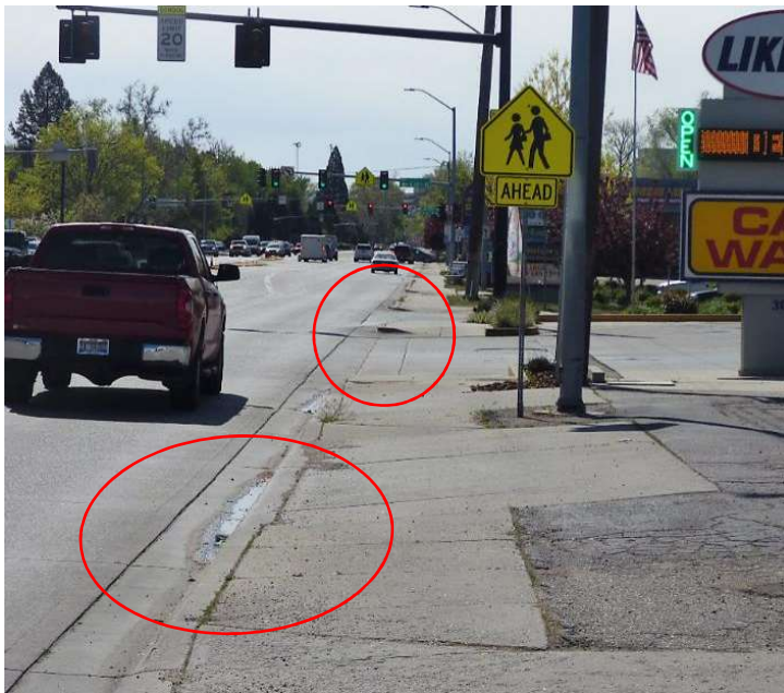
Sidewalk with multiple access points, loose gravel, deteriorated crosswalk striping, and little physical separation from heavy traffic
