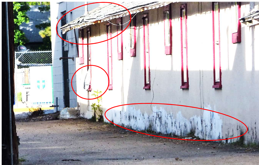
Deteriorating roof, walls/paint, fascia, windows
