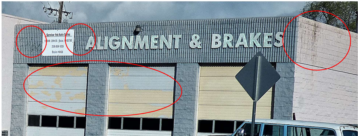
Deteriorating upper walls/parapets, bay door paint, signage; evidence of roof drainage problems
