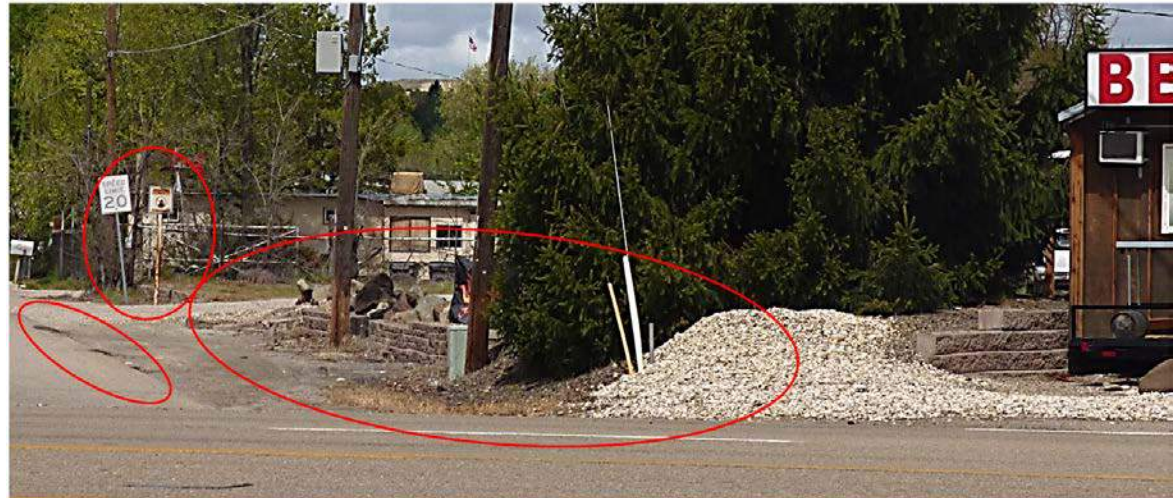
General site maintenance issues; lack of curb/gutter, deteriorating signage, gravel lot, etc.
