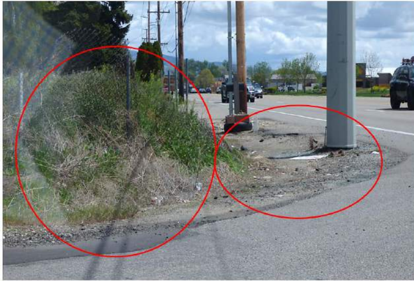
Deteriorating street, no sidewalk, no curb/gutter, weeds, drainage/erosion issues
