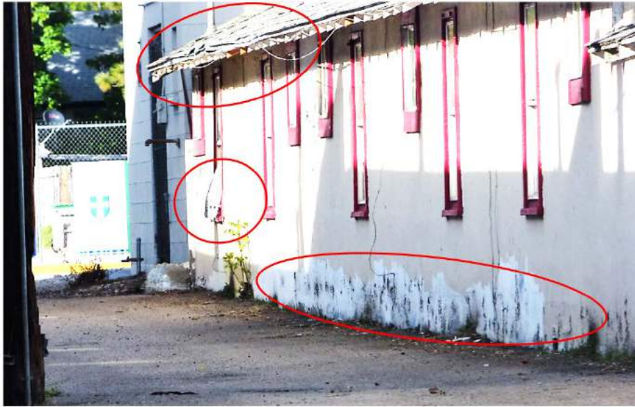
Deteriorating roof, walls/paint, fascia, windows
