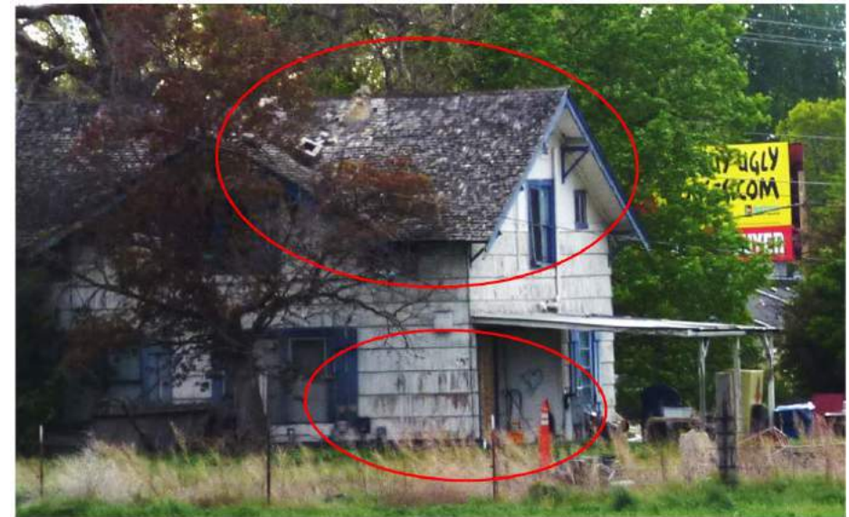
Extensive roof damage, deteriorating siding, paint, shutters, etc.
