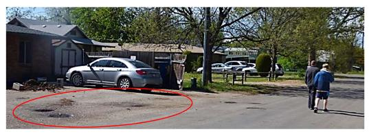
No curb/gutter, gravel driveway, potholes, drainage problems; no sidewalk/pedestrian safety
