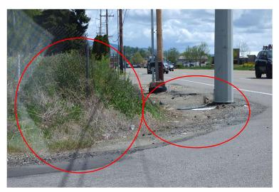
Deteriorating street, no sidewalk, no curb/gutter, weeds, drainage/erosion issues
