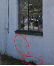
Deteriorating masonry, paint, bay doors; evidence of foundation problems
