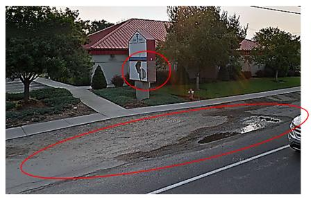
Sign damage, deteriorated street margin, drainage problems
