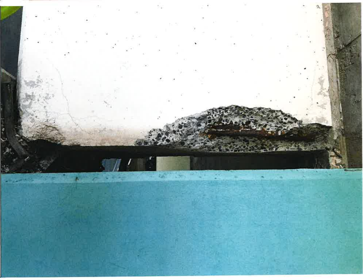
West face of the beam end. One stirrup was exhibiting corrosion. The concrete beneath these stirrups was sound.
