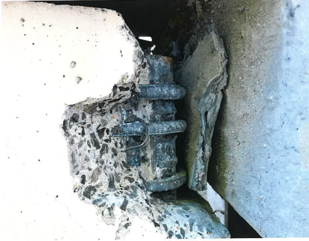
Example of a beam bearing pad replacement. After shoring, the entire bearing surface is demolished up to the #14 longitudinal bar so that a new pad can be inserted.
