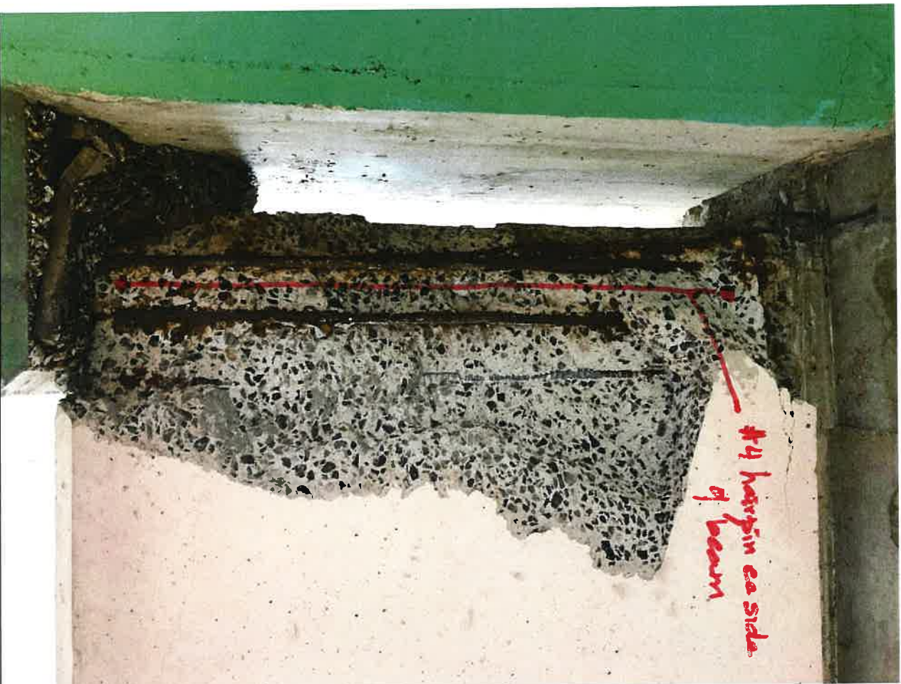
East face of the beam end. Two stirrups and part of another were exhibiting corrosion. The concrete beneath these stirrups was sound.
