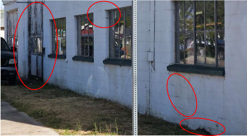
Deteriorating masonry, paint, bay doors; evidence of foundation problems
