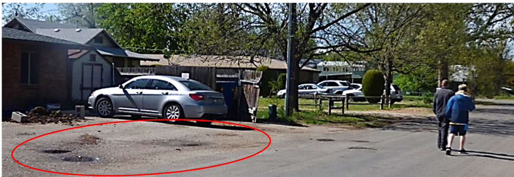
No curb/gutter, gravel driveway, potholes, drainage problems; no sidewalk/pedestrian safety
