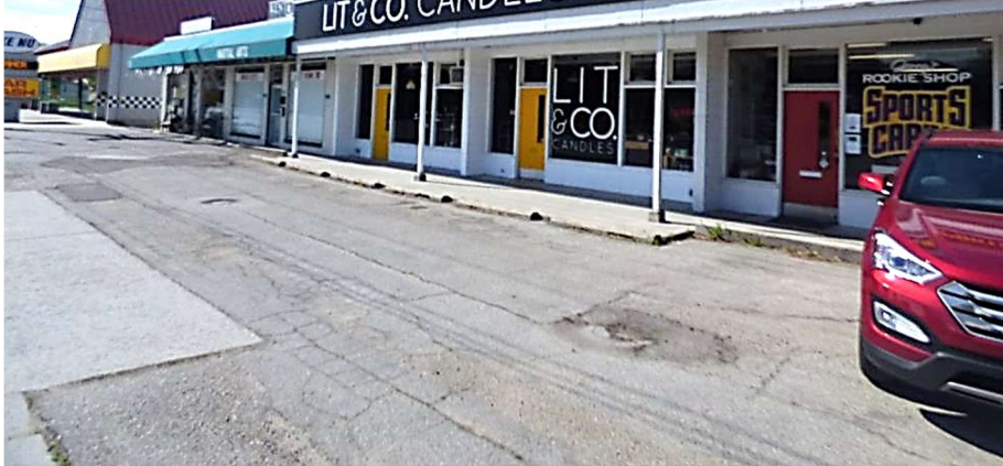
Deteriorating parking surface with faded/missing space markings
