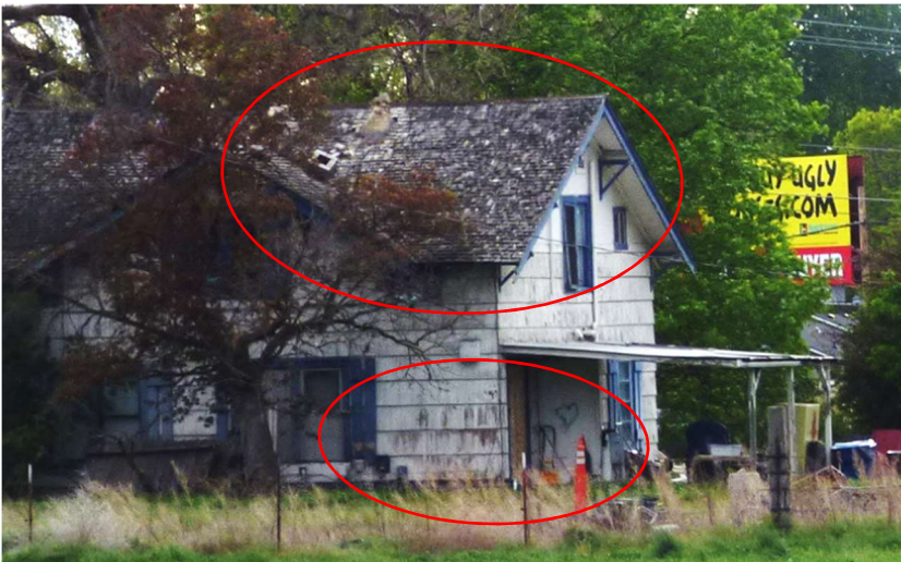
Extensive roof damage, deteriorating siding, paint, shutters, etc.
