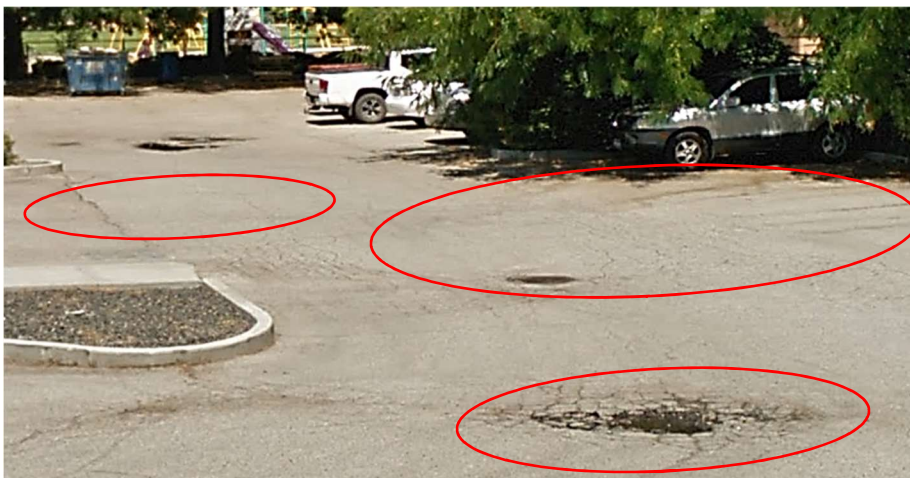
Deteriorating parking surface with faded/missing space markings
