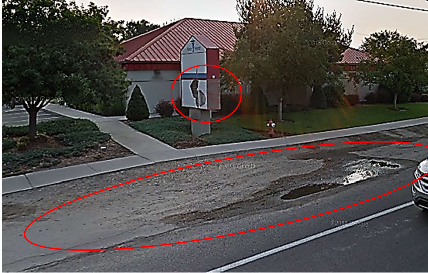
Sign damage, deteriorated street margin, drainage problems
