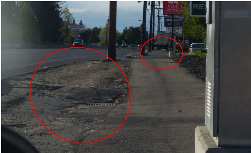
Badly deteriorated street margin, no curb/gutter; sidewalk area used for truck parking
