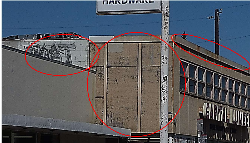
Deteriorating exterior walls/siding, paint, signage; rusted roof flashing
