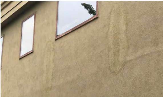
Moisture damage to a building exterior on West Overland Road
