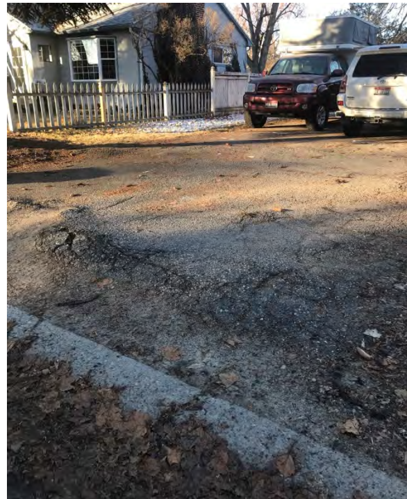
Buckling driveway along South Berkeley Street
