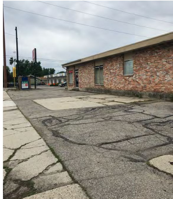
Cracked and patched parking lot on West Overland Road
