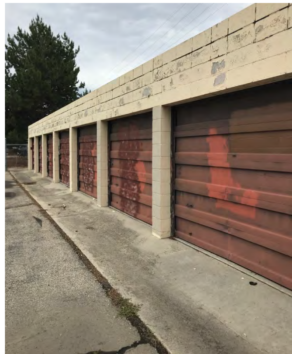
Deterioration of cement block building on West Overland Road
