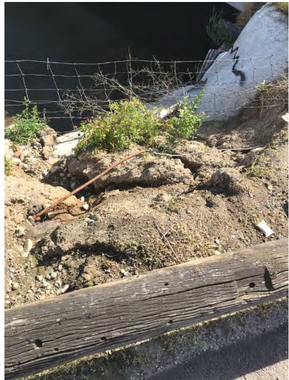
Canal opening along South Vista Avenue. Wire fence is an inadequate barrier to entry, creating an unsafe condition. The bottom picture shows a rusted protruding piece of rebar, which creates an injury risk.
