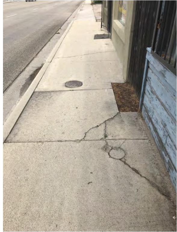
Narrow sidewalk directly adjacent to a travel lane on West Overland Street between South Gourley Street and South Hervey Street. Current pedestrian safety guidelines recommend a minimum five-foot buffer between traffic and pedestrians.
