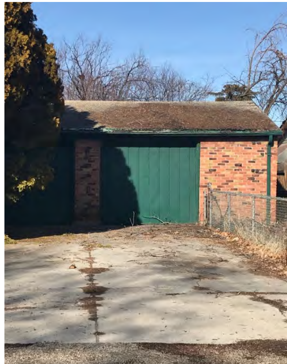
Deterioration of roof on West Clinton Street.
