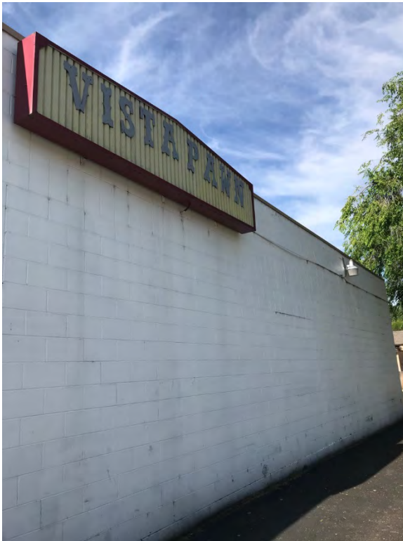
Pocked and deteriorating cement block wall with peeling paint on South Vista Avenue.
