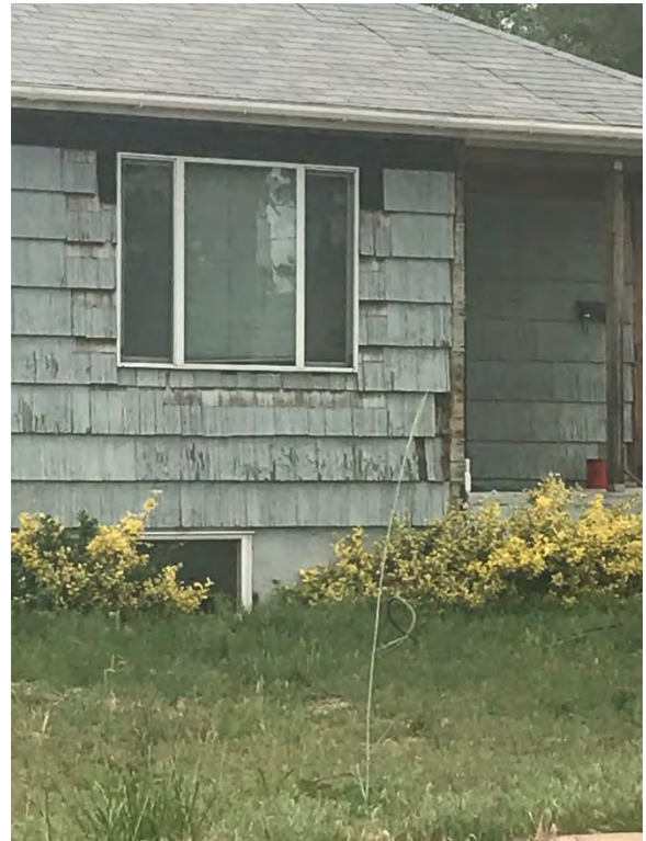
Deteriorated wooden siding on South Victoria Drive
