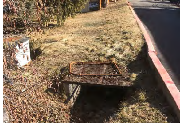
Drainage infrastructure adjacent to North Latah Street does not adequately prevent falls, injury, or entry.
