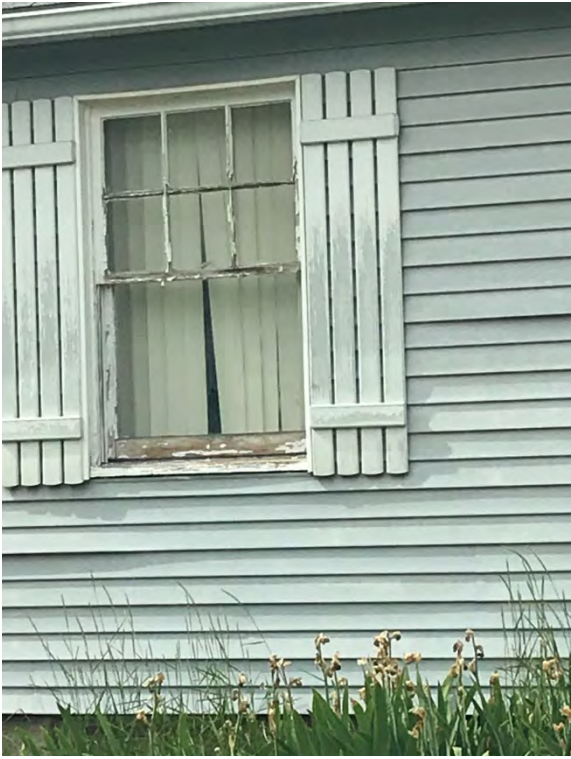
Deteriorated wooden window casing and siding on West Ponderosa Road
