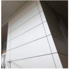
Metal Panel: Skycore Style: Skycore Color: Silversmith Pattern: Composite, dry joint
