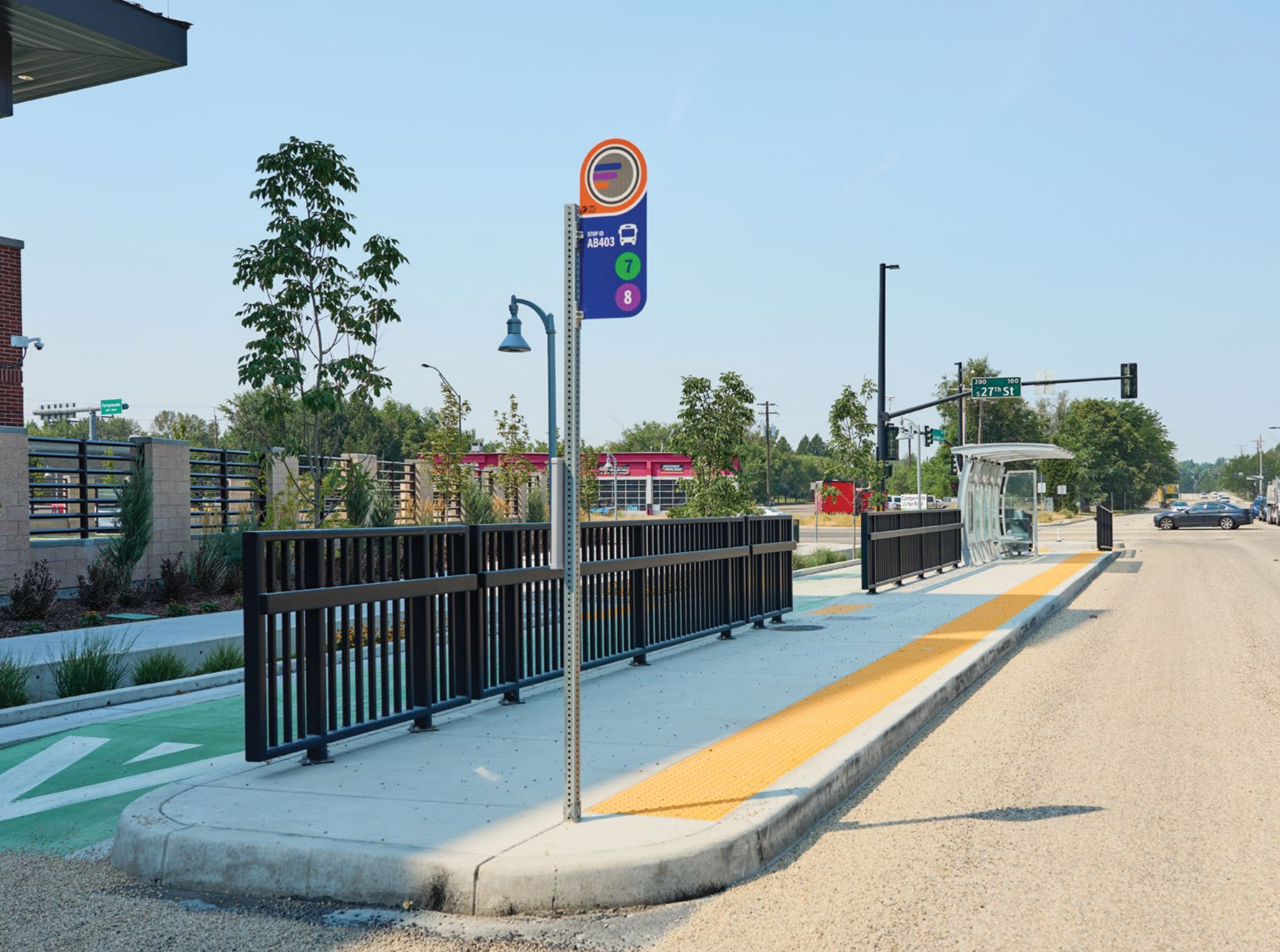
New transit station at 27th Street and Fairview Ave.
