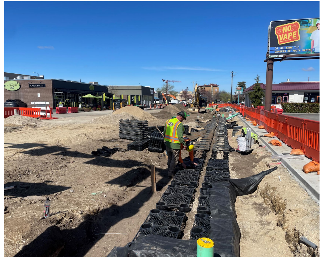
1500 Block, Current Status
