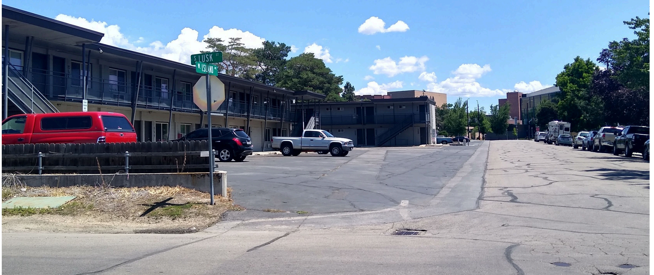
Current Status of Project Site at Island Ave. & Lusk St.
