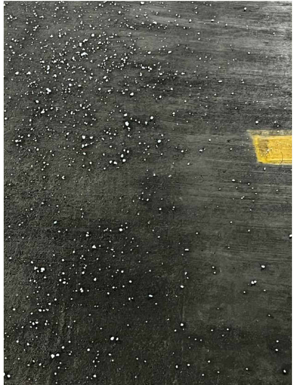
Photo of level 3 of the garage. This level was not coated with a traffic membrane. Granular deicing salt is spread onto the deck during freezing weather.
