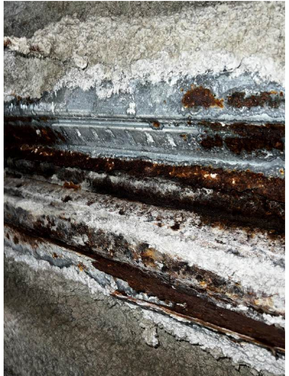
The chloride solution causes corrosion of the mild-steel panderk. Hidden by the insulation, the corrosion proceeds until the metal deck is severely corroded. The corroded metal panderk breaks loose exposing the concrete above.
