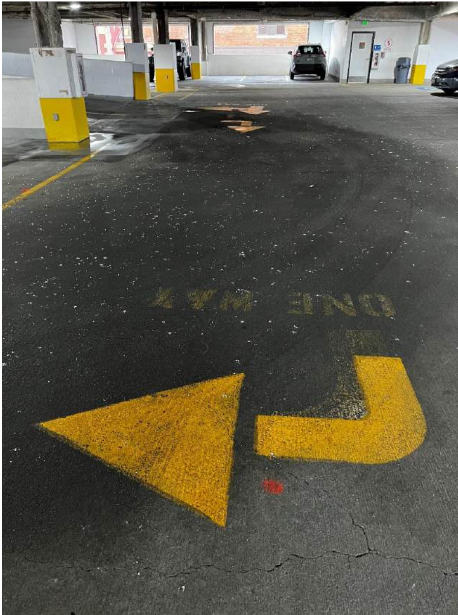
Photo of level 3 of the garage. This level was not coated with a traffic membrane. Granular deicing salt is spread onto the deck during freezing weather.
