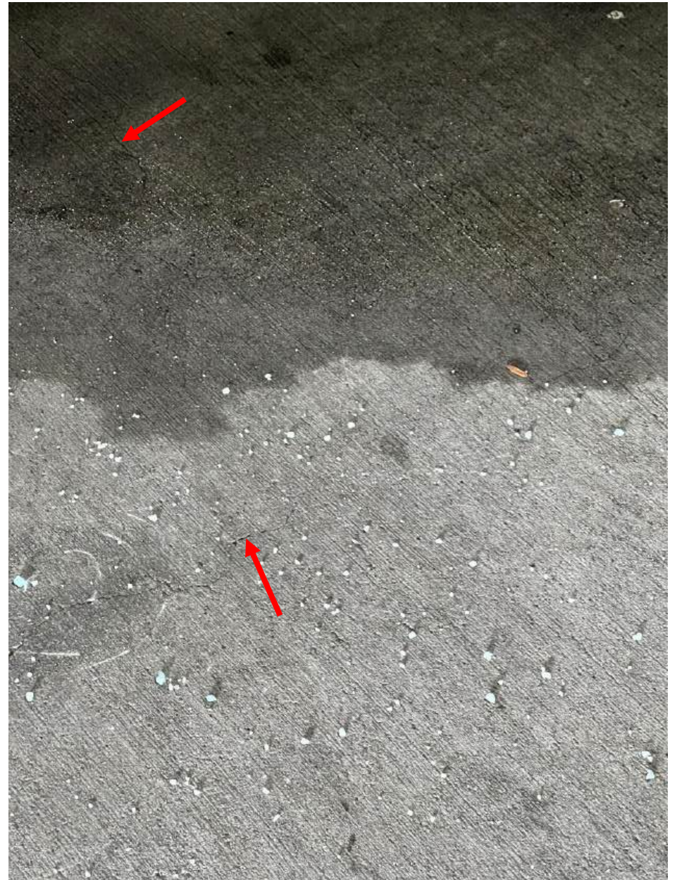
The granular salt dissolves into the standing water and enters the concrete, particularly through cracks (red arrows).
