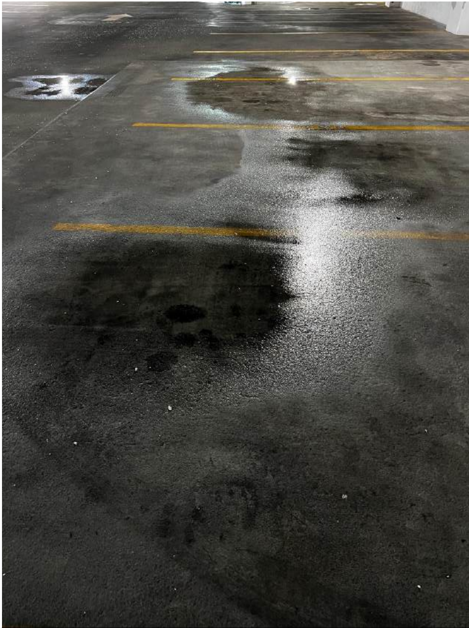
Melted snow or rain water entering the garage directly or carried in by vehicles puddles on the deck.
