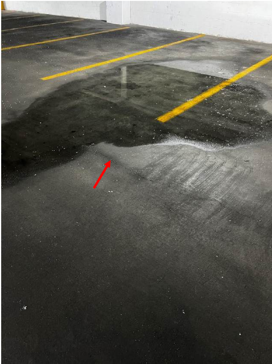
The granular salt dissolves into the standing water and enters the concrete, particularly through cracks (red arrows).
