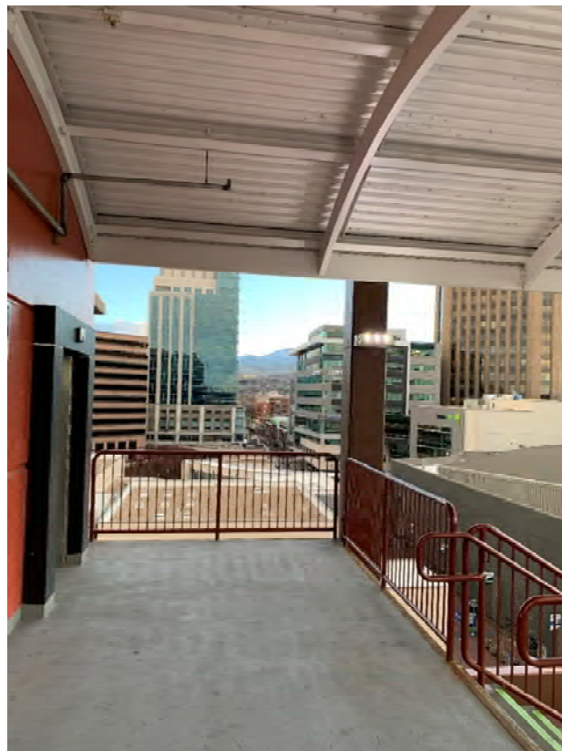
East Stairway, 8 th Floor, looking north.
