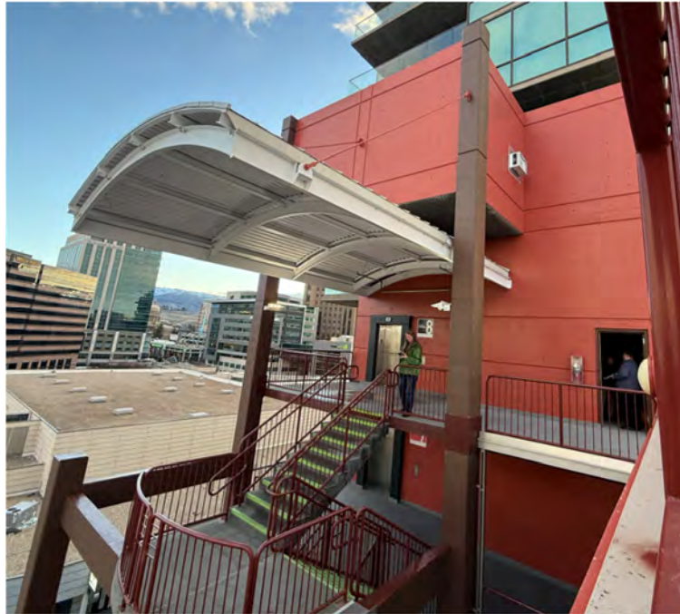
West Stairway, 8 th floor, looking northeast.
