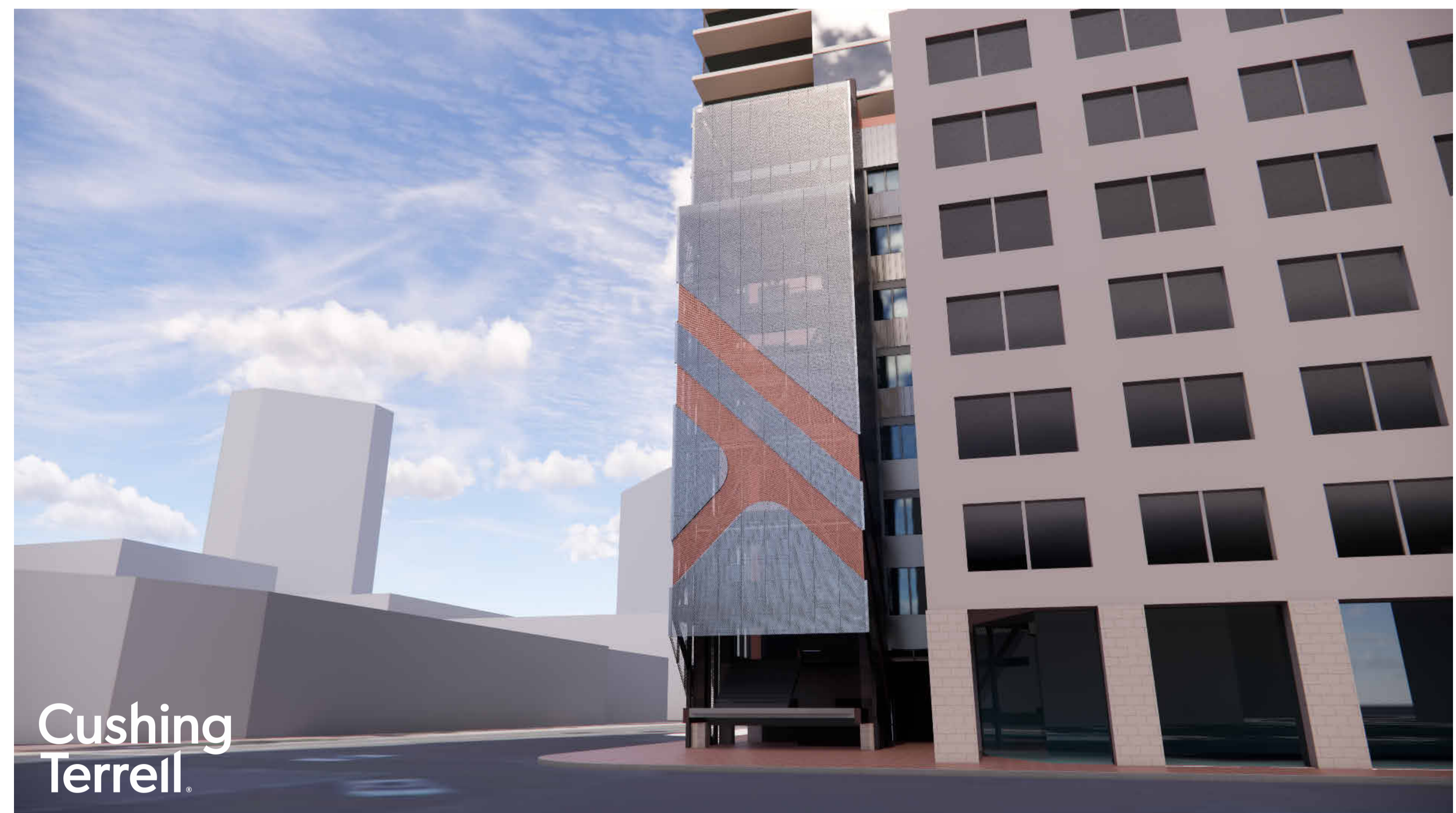
WEST TOWER GROUND FLOOR LOOKING EAST
