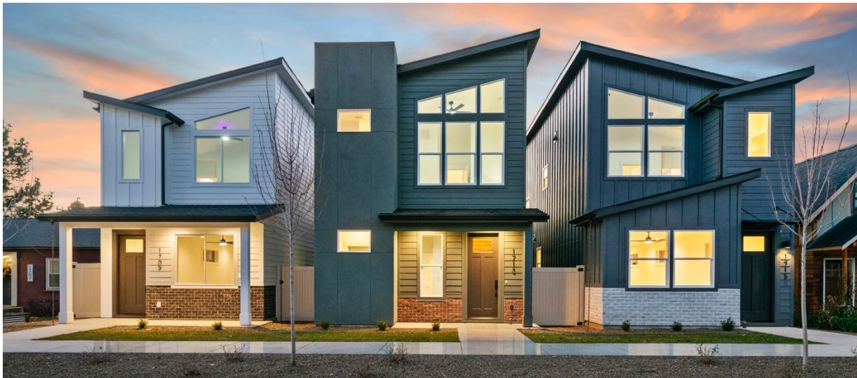
Completed 1711 N. 31st Street Residential Development
