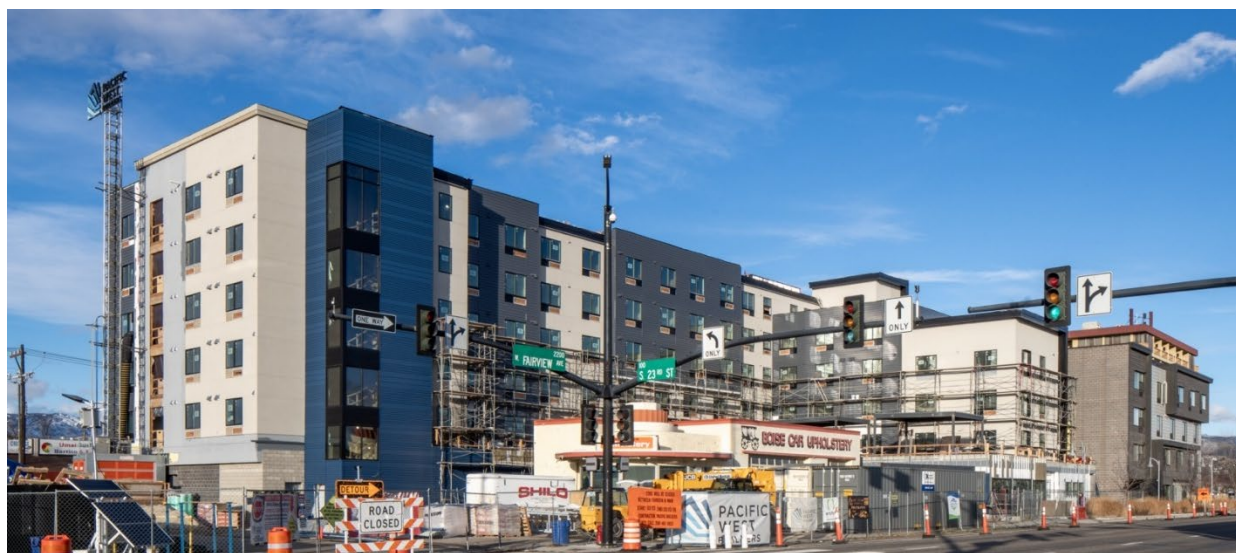
New Path 2 under construction
