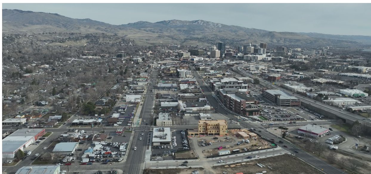
Aerial view of the 30th Street District where The Finch, a Type 1 Participation Program partnership with Roundhouse, is currently under construction
