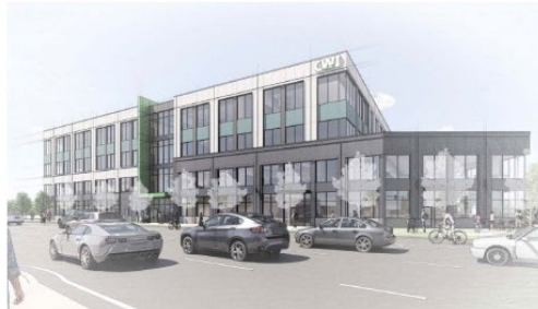
View of building, taken from Main Street and looking northwest.
