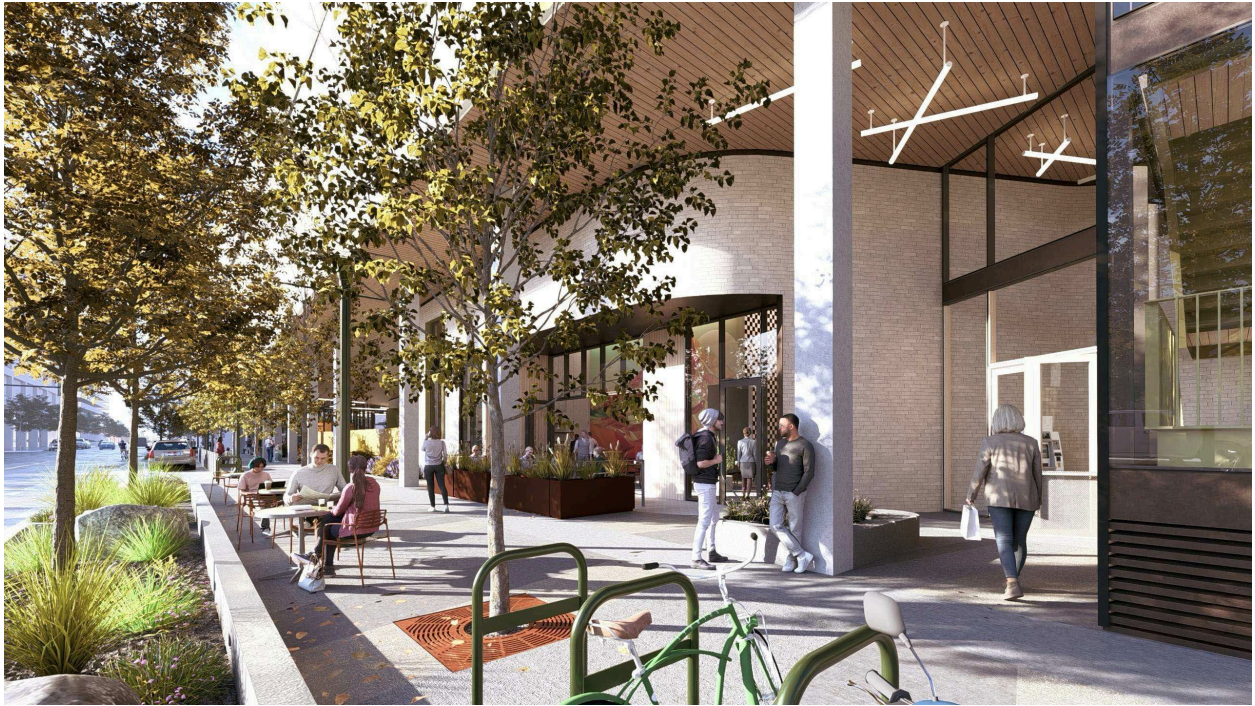
View of ParkBOI stair entrance and commercial unit near the corner of Jefferson Street and 10th Street
