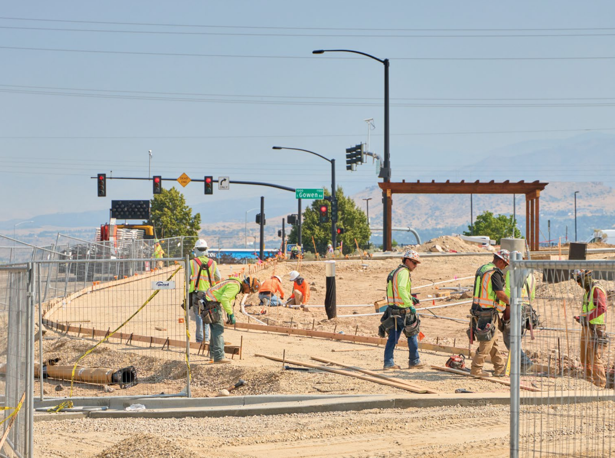
Construction of Maverik, a Type 1 Participation Program project. The Maverik will be a convenience store and fuel station located at the corner of Eisenman Road and Gowen Road.
